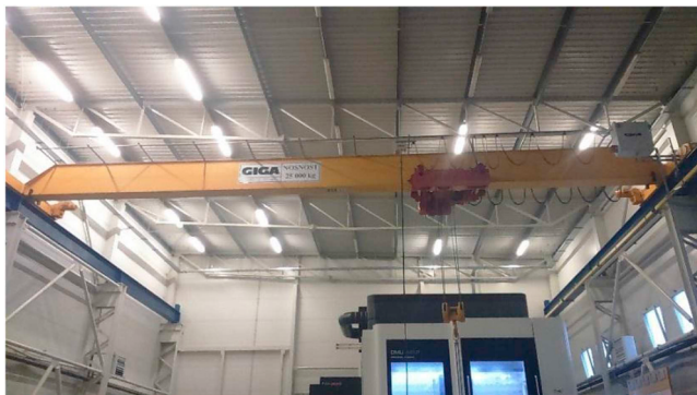
Fig. 1. Current state of illumination in the manufacturing hall.
