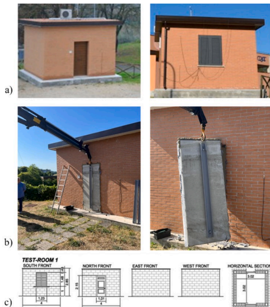
Fig. 3. a) Test room, b) removal stage of one of the panels, and c) facades and plan of the testroom (pictures from [53]).
